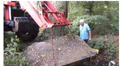
Photo - Lifting the slab
