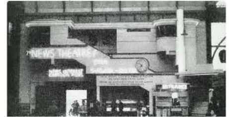
6 Exterior showing the steps up to the entrance into the auditorium
