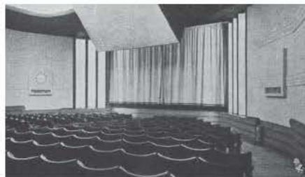
3 Interior of the Waterloo cinema showing the box section through which the projected beam passes to the screen 1
