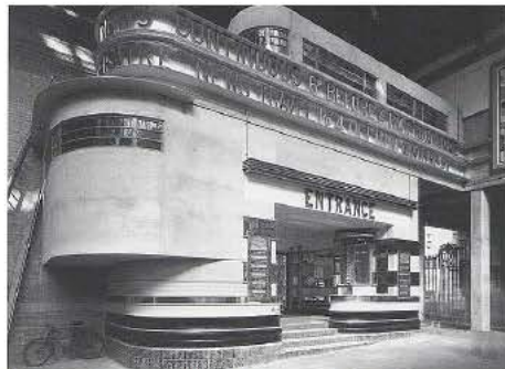
Victoria Station News Cinema when first opened in 1933 1 Closed 1981
