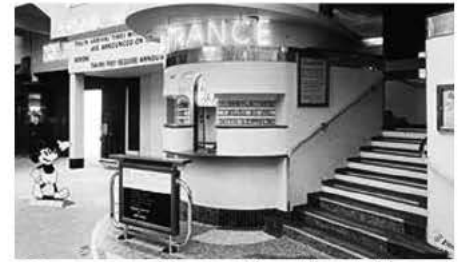
5 Entrance and steps with a pillar visible at the rear left
