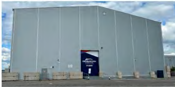
Massive concrete blocks surround the stage - photo FIS
